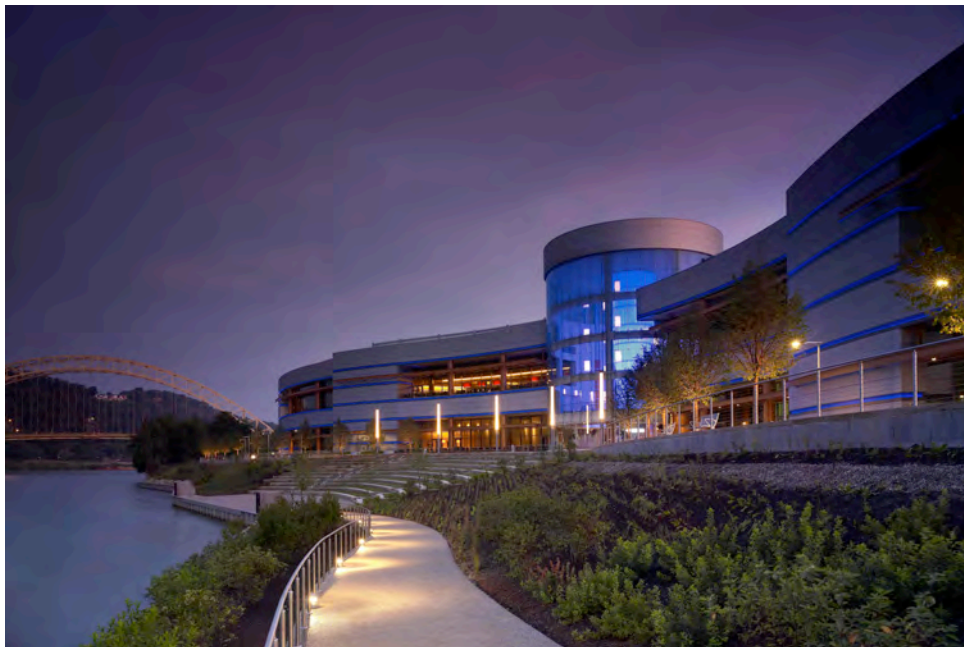
The Rivers Casino replaces a former steel factory and adds a new destination along a riverfront park that has revitalized Pittsburgh's North Shore. Photo © 2009 Brad Feinknopf
