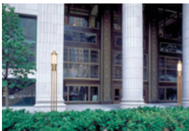
Philadelphia's The Wanamaker Building is being transformed into a Macy's store.
