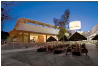
The Shops on Lake in downtown Pasadena, California, is anchored by Macy's.
